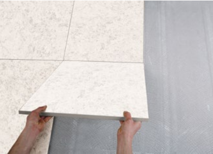
ADHESIVE INSTALLATION ON FOOTING
